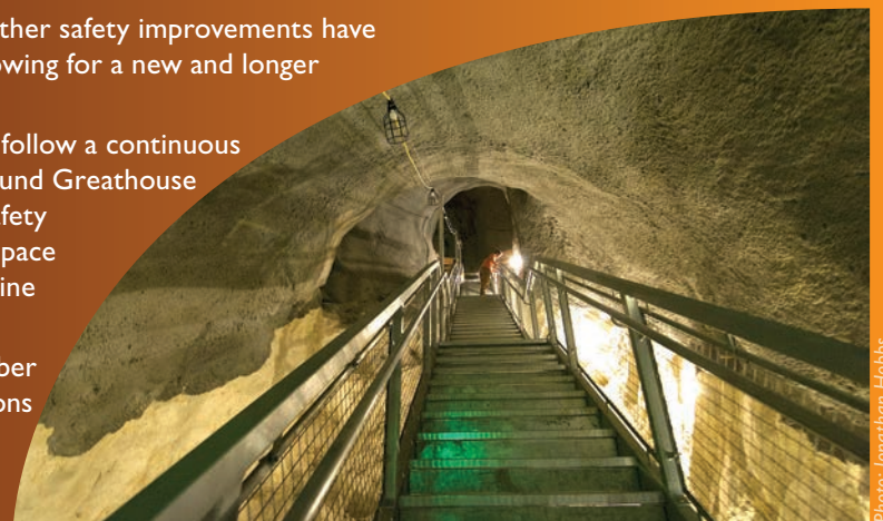
New underground stairway.
